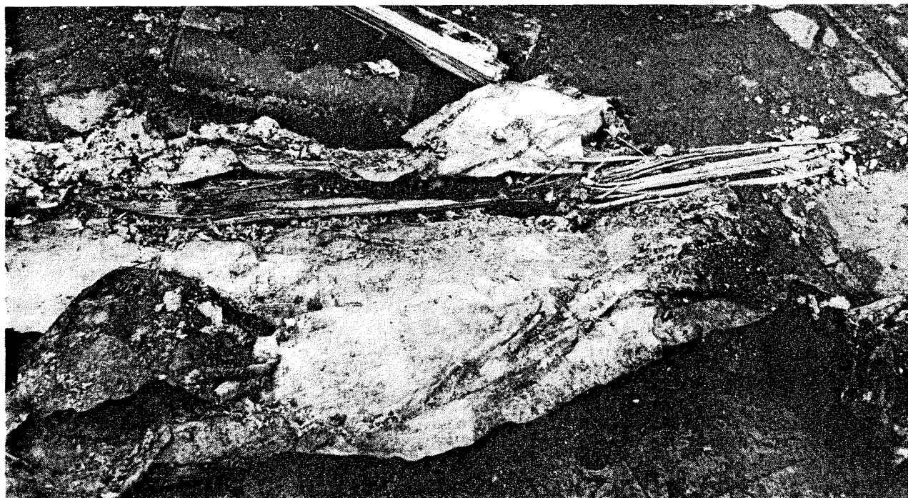
Figure 7. Splintered remains of the wooden floor.
