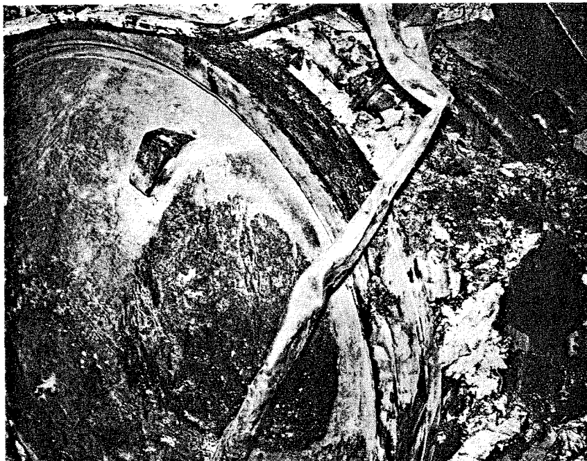
Figure 5. View of the cover (top) of the main condenser.
